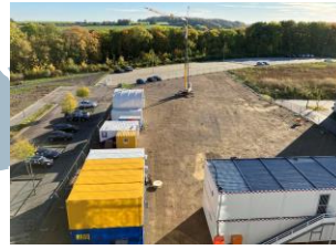
5G for construction
