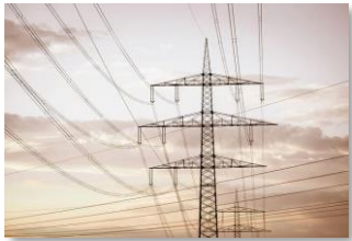
5G for energy monitoring
